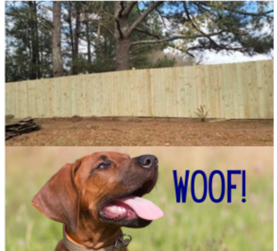
Hurray for cool weather! Our crew isn't constantly mowing and responding to hurricanes, so we can get projects done - like this new perimeter fence at our TransPUptation Center . Thanks for making it possible!
